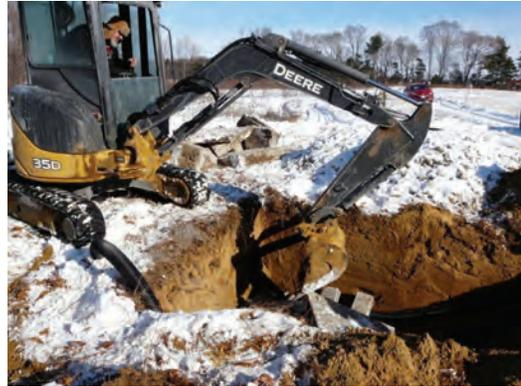
**3. Fill with Rubble** – Place rocks, concrete rubble, logs, timber, blocks and/or bricks to create chambers at different depths with connecting passageways. The snakes should be able to move throughout the structure to find their preferred wintering microhabitat. Do not use railway ties or pressure-treated lumber.
